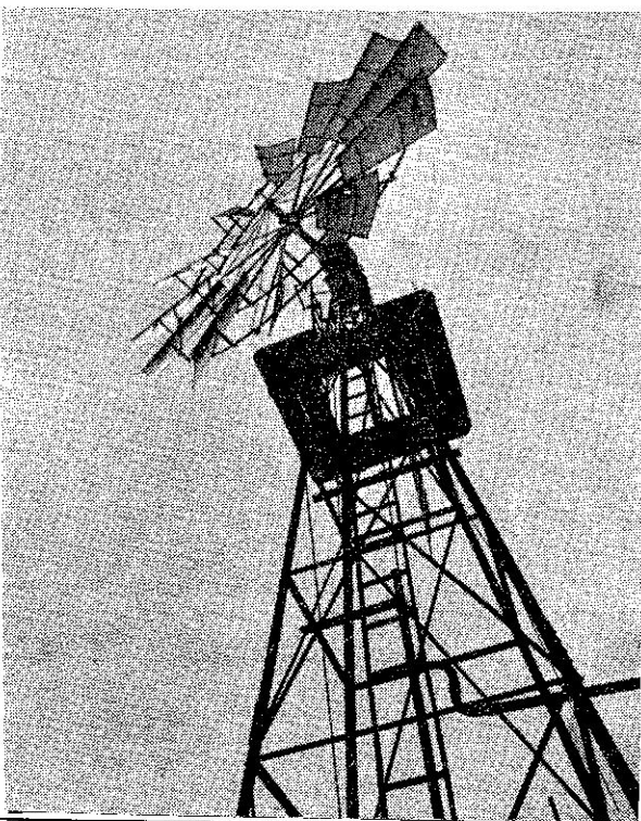
Fig. 5. Type WP-II deep well windpump developed by the National Aeronautical Laboratory, Bangalore.
