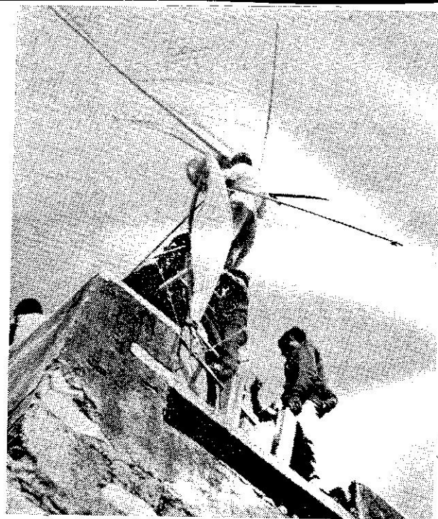
Fig. 6. Deep well windpump built by village artisans, designed by Marcus Sherman.
